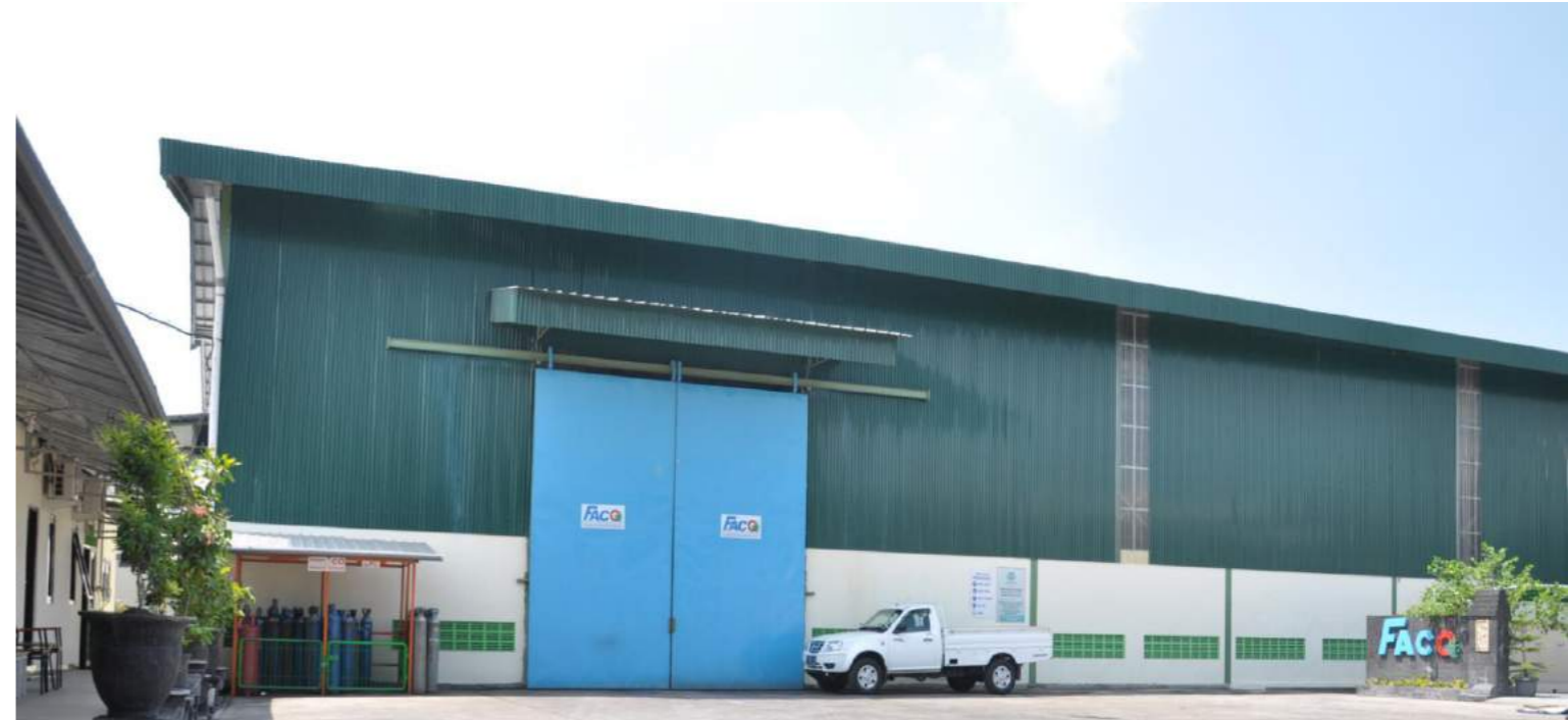
Fabricate & Sand Blasting Painting 6000 M 2 , kapasitas hoist crane 20 Ton
